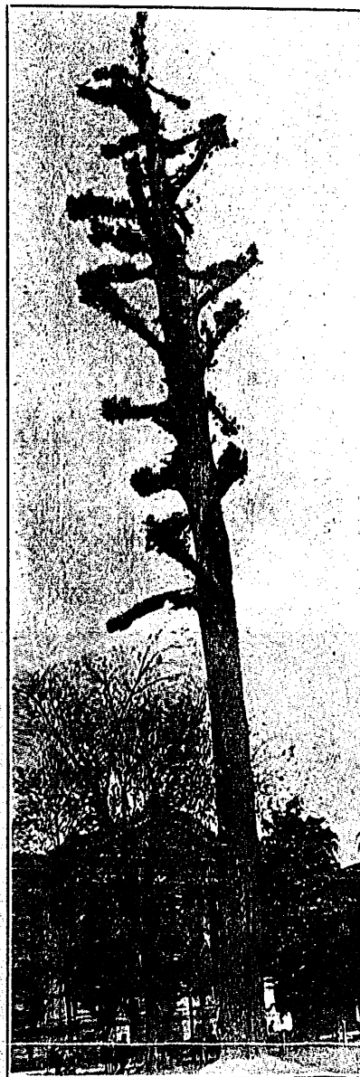
Mr. Virgin very artfully interlaced and spliced the roots of the tree to its trunk, performing a most unusual operation.
